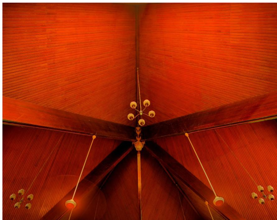
**Figure 1** Slanted glued-laminated beams used as load bearing roof components in FRIM's mosque while exposing their beauty
