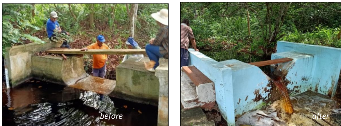
Figure 5 Check dam maintenance and redesign to v-notch shape at Parit Pulai check dam
