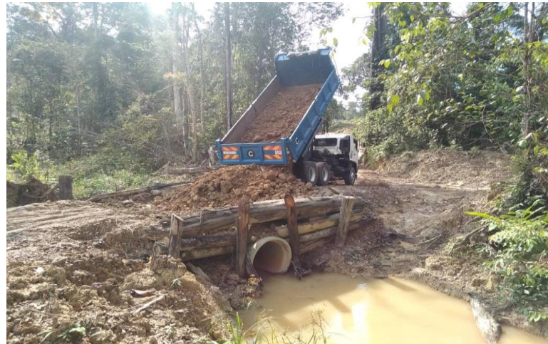
Figure 1 Forest Bridge made of log stringer
