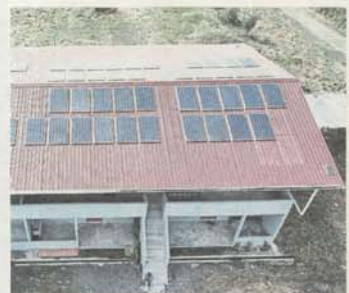
A household in rural areas generally requires 2,000 watts of solar panels, which cost RM7,500 without the battery
