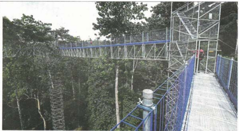
The 250m-long aluminium Forest Skywalk in Kepong Botanical Garden is an environmentally-friendly structure with safety features. — Photos: Bernama
