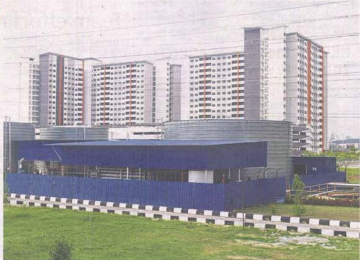
The plant is currently distributing 5MLD to industries nearby through underground pipelines.
