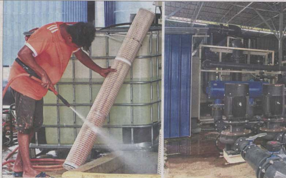
The purified water from the water reclamation treatment plant is used to clean its filters. (Right) It is also stored in the drum at the plant to clean the ultrafiltration system. — Photos: SAM THAM and MOHD SHAHRIL ROSLI/The Star
