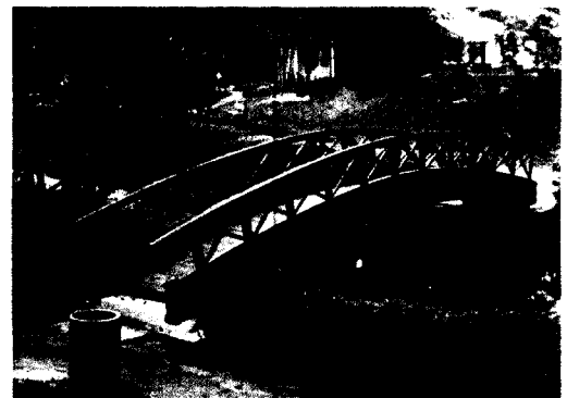
Figure 5 Glulam footbridge at FRIM
