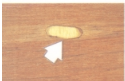
Figure 10. Large worm hole - worm hole more than 1.5 mm in diameter or a channel made by a wood borer. This includes holes made by marine borers
