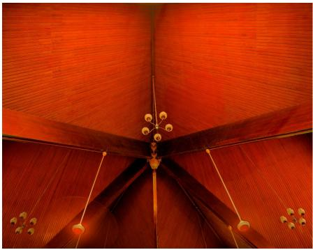
Figure 1 Slanted glued-laminated beams used as load bearing roof components in FRIM's mosque while exposing their beauty
