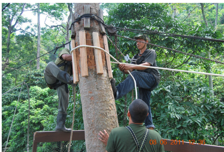
Figure 7 A sufficient and orderly placements of spacer blocks to keep the cable and rope separated from the bark
