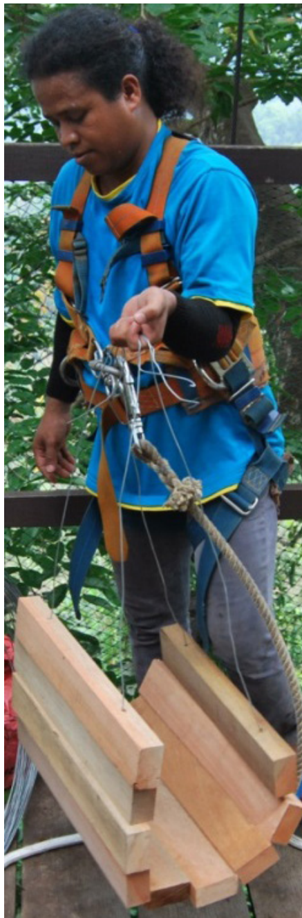
Figure 6 Spacer blocks are fasten together using wires to simplify the installation
