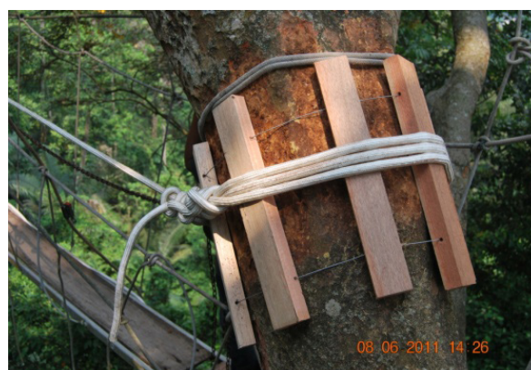
Figure 8 A set of spacer block was replaced with a new timber at different positions to avoid further damage of the bark
