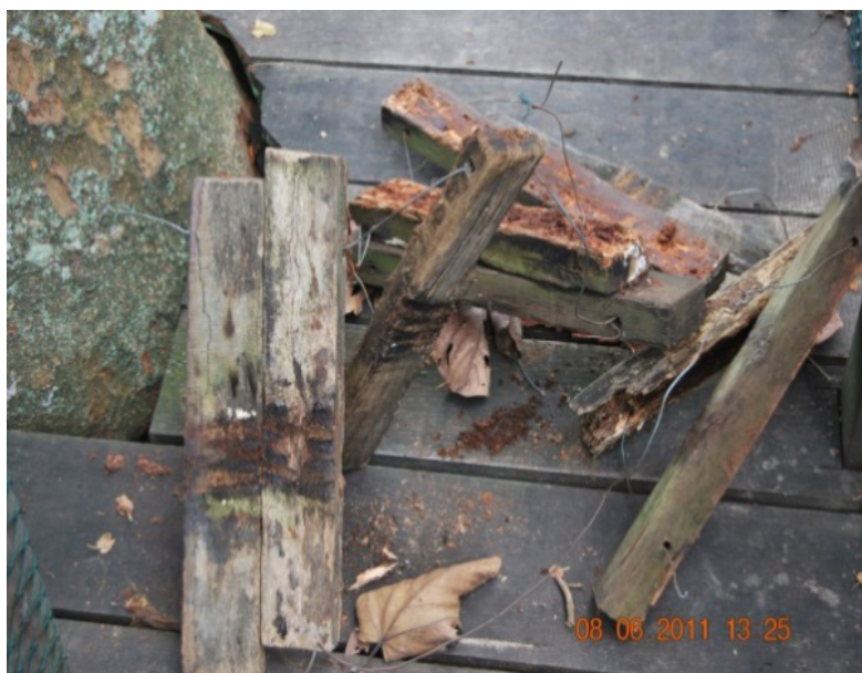
Figure 5 Damaged blocks as a result of both biological deterioration and mechanical force
