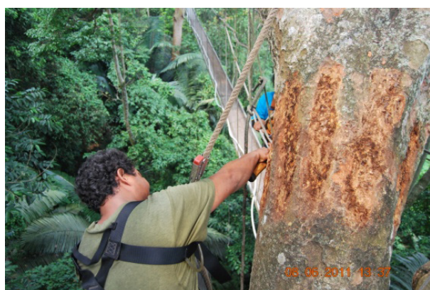
Figure 8 A set of spacer block was replaced with a new timber at different positions to avoid further damage of the bark
