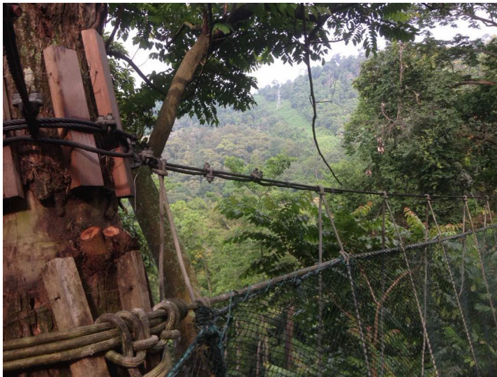
Figure 2 Metal cables and polyester ropes tied around sets of spacer blocks
