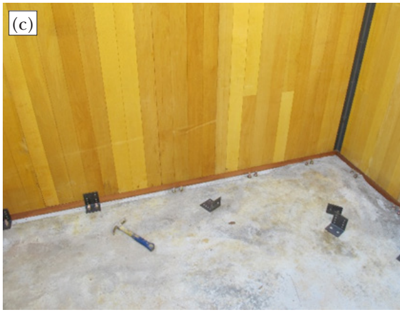
Figure 3 Erecting CLT panels with appropriate connectors, (a) first set of CLT panels erected, (b) erecting process of CLT panels, (c) angle cleats and raw bolts were used to hold the panels to the floor and (d) vertical angle bars were used to hold panels at each corner
