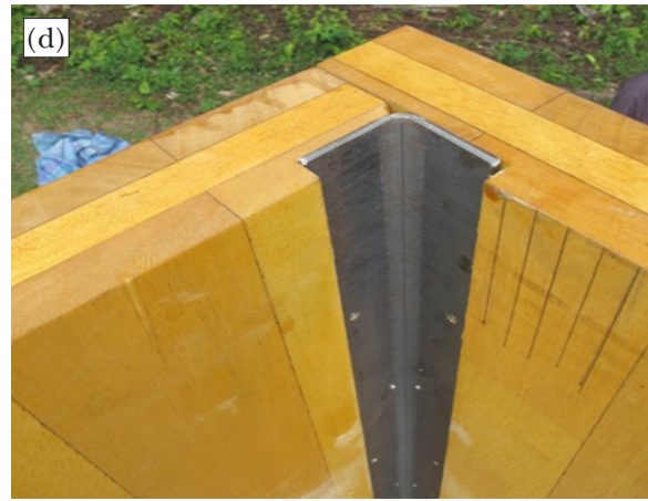
Figure 3 Erecting CLT panels with appropriate connectors, (a) first set of CLT panels erected, (b) erecting process of CLT panels, (c) angle cleats and raw bolts were used to hold the panels to the floor and (d) vertical angle bars were used to hold panels at each corner
