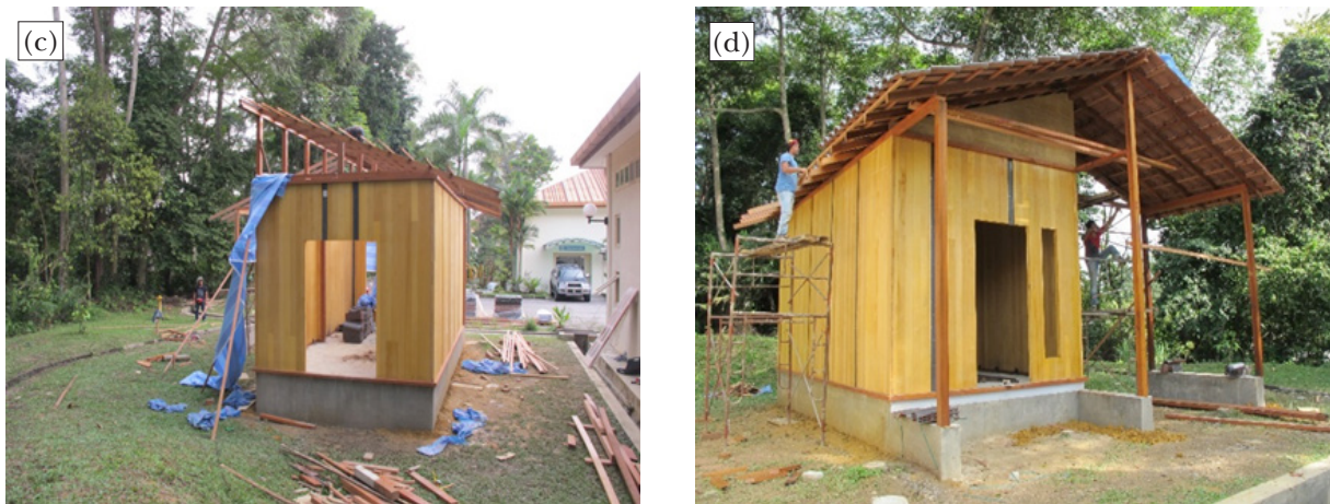
Figure 4 Fabrication of the roofing system, (a) the installation of mono-pitched roof, (b) roof tiles installation in progress, (c) rear view of the CLT structure during construction and (d) semi finished CLT structure
