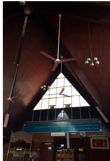
Figure 4 The interior of Masjid Jamek FRIM - roof rafters made from Glulam beams
