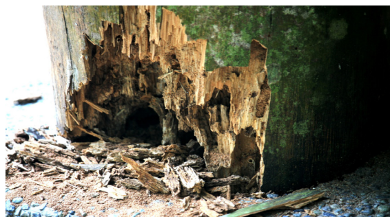
Figure 1 Sample of a pole attacked by fungus
