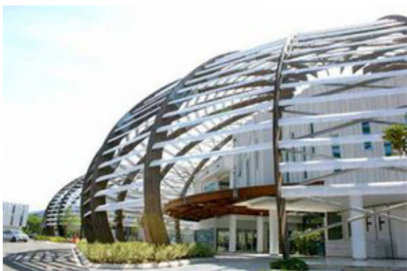
Figure 12 Curved glulam beams were used as the dome hovering design of the Crops for the Future Research Centre (CFFRC), University of Nottingham, Broga, Selangor, Malaysia
